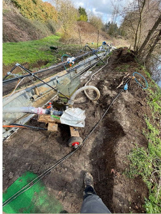
Figure 96: March 2023 - prototype in the trench
