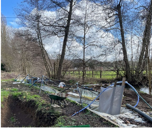
Figure 94: March 2023 - prototype in the trench
