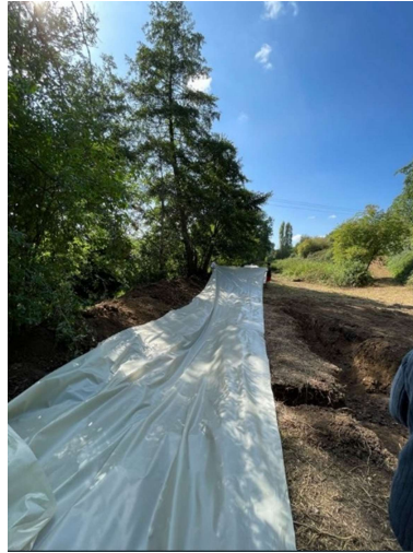
Figure 19: Laying the tarp in the trench
