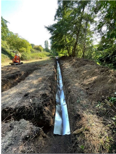
Figure 20 : Installation of the foam protection in the trench
