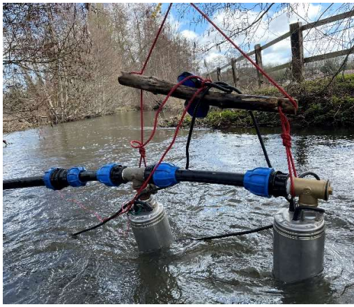
Figure 95: March 2023 - 2 pumps installed in the river
