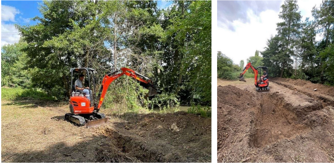
Figure 17 : Photos of the trench and tank excavation
