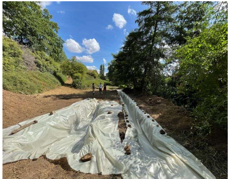
Figure 18 : Installation of the tarp in the tank and final rendering
