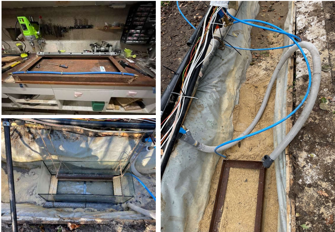
Figure 85 : Phots of the metal made armatures
