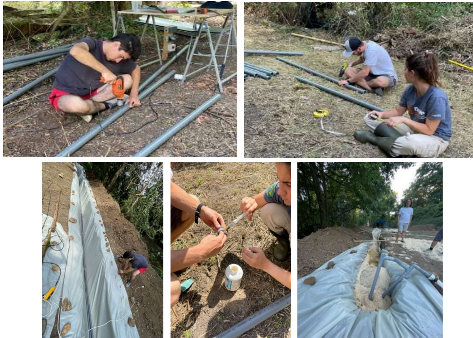
Figure 22 : Drilling of injection holes, gluing of PVC fittings and rendering
