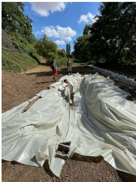
Figure 20 : Installation of the foam protection in the trench
