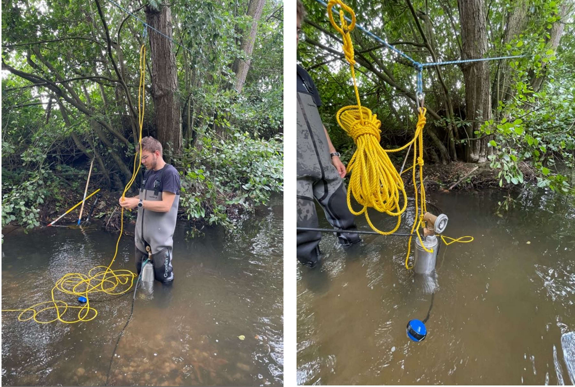
Figure 24 : Installation of the pump in the river
