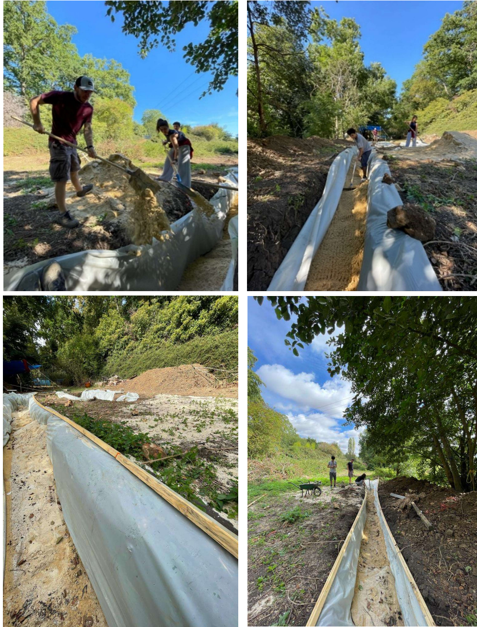
Figure 23 : Filling the trench and pulling the tarp
