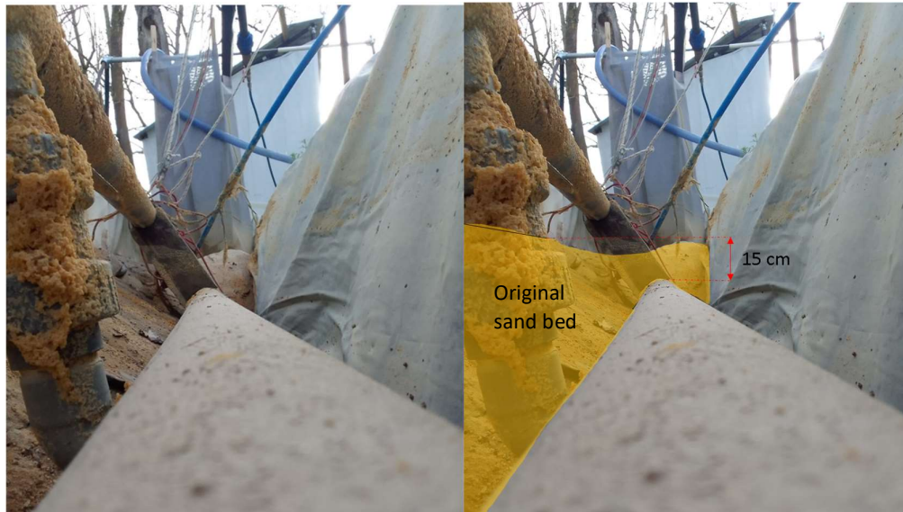
Figure 99: view of the pipe sunk in the trench
