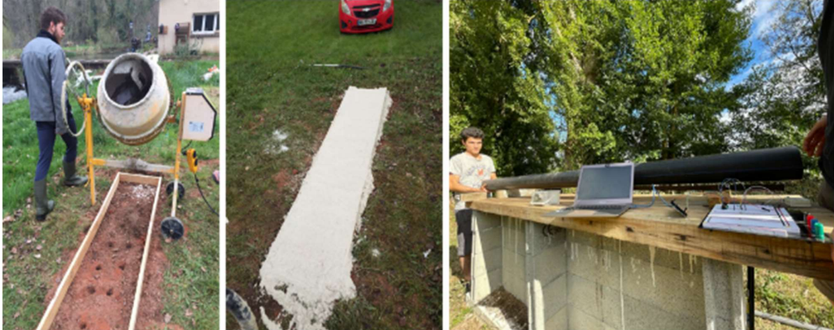
Figure 27: Construction de l'établi
