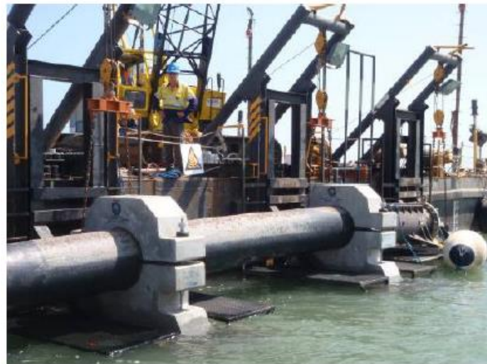
Figure 14 Installation of several concrete weights simultaneously
