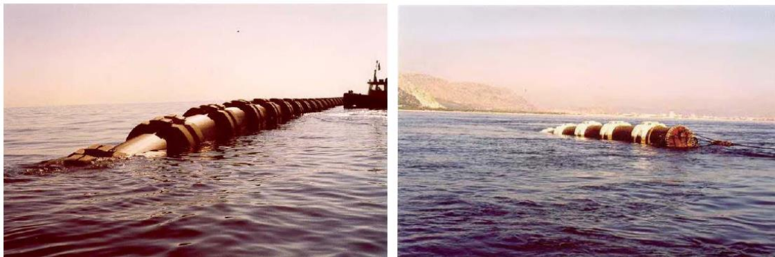
Figure 3 Initiation (left) and End (right) of pipe section installation.
