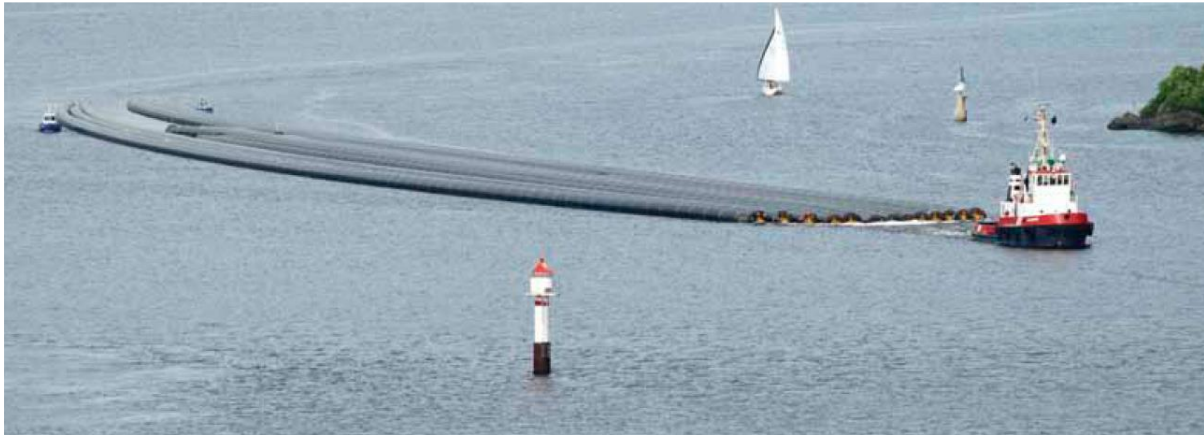
Figure 1 Pipe sections towing to construction site.
