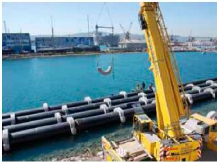
Figure 13 Installation of concrete weights using crane (left) and frame (right)
