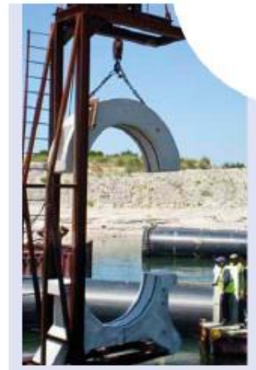
Figure 13 Installation of concrete weights using crane (left) and frame (right)
